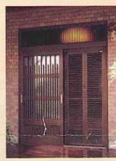
玄関引戸取替
